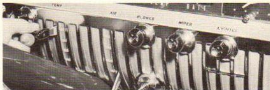
Heating and ventilating controls
