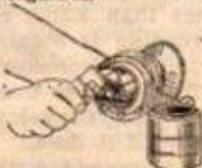
Figure II.—This illustration shows position of wrench after lock-nut has been loosened.
